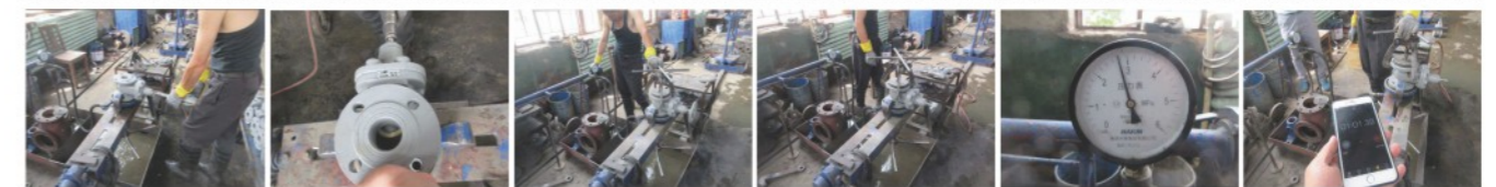
Open/close valve 5times | Open/close valve 5times | Fixed the valve | Beginning test | Set 2.4Mpa | Keep 60s
